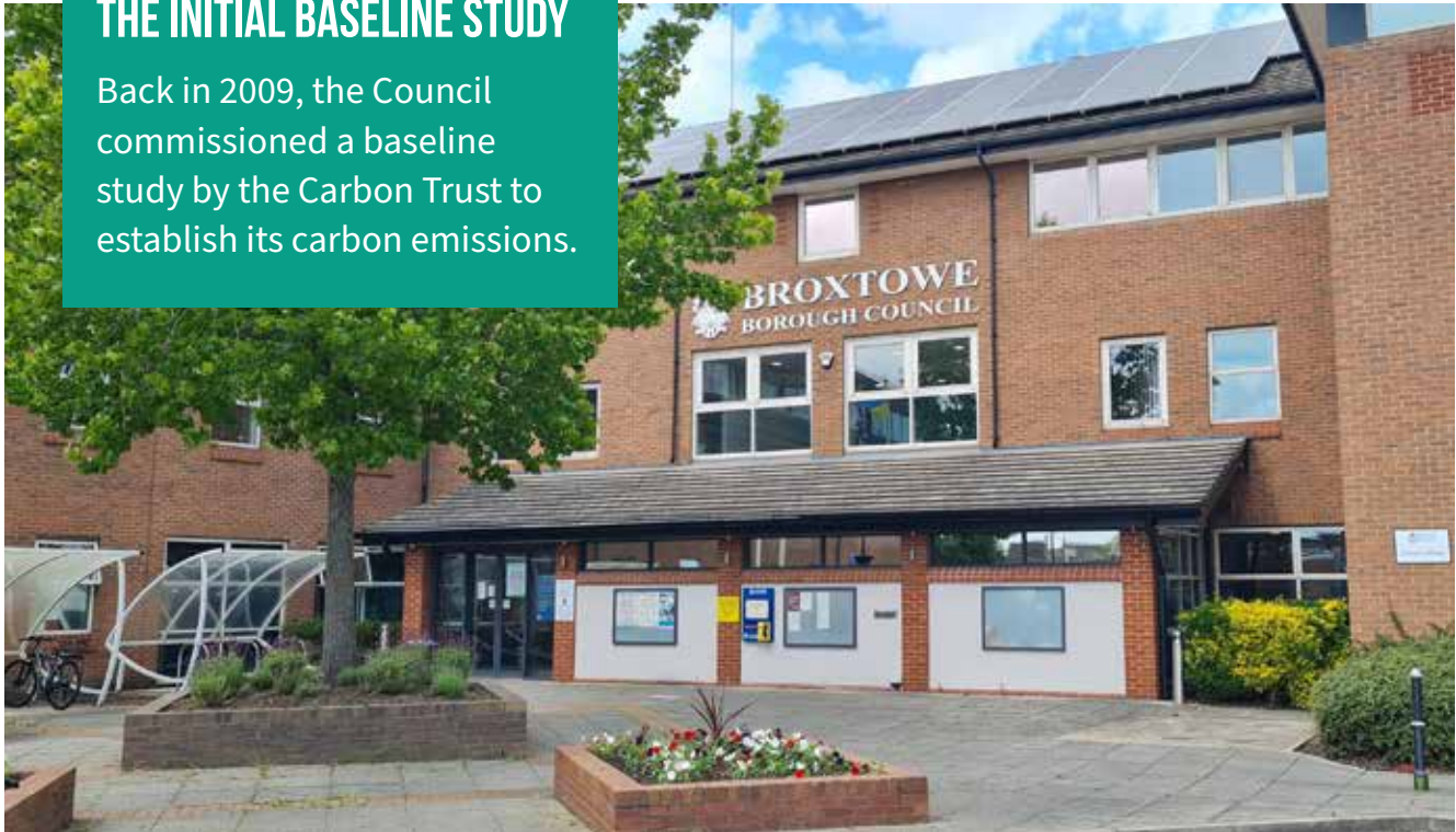
Image 3: Solar PV on the main Council offices at Foster Avenue - Beeston
