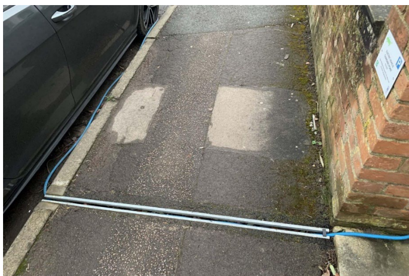
Figure 8: Example of electric vehicle cable channels for off street EV charging.
