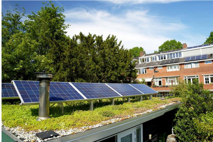
Figure 4: Example of a biosolar roof
